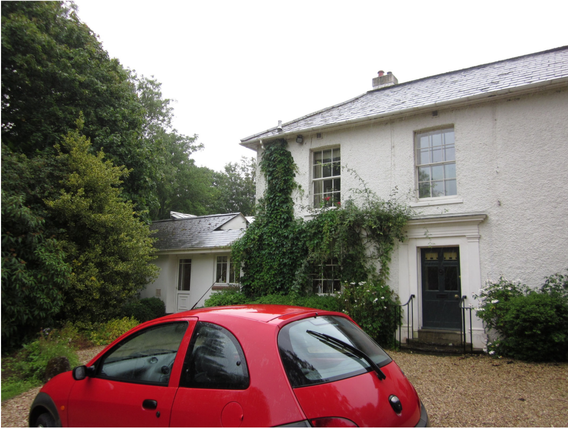
North elevation, main house and east extension
