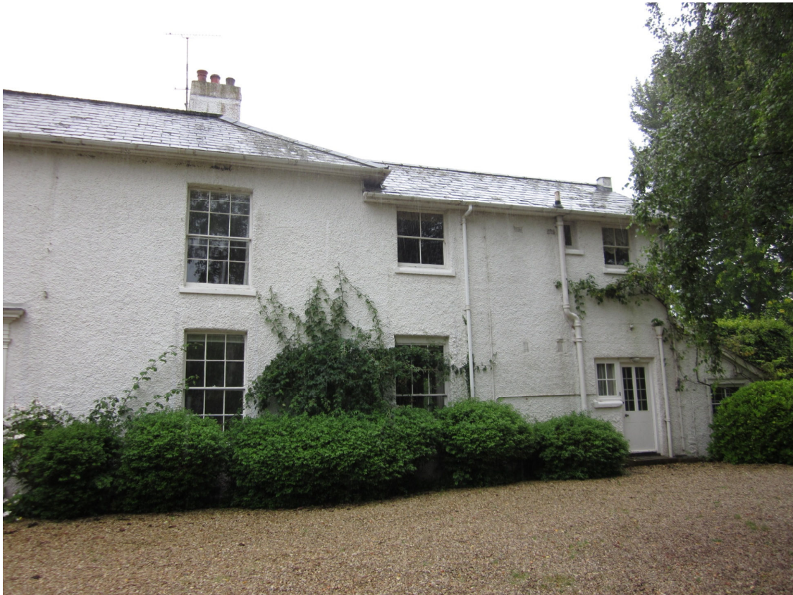
North elevation, main house and service (west) wing
