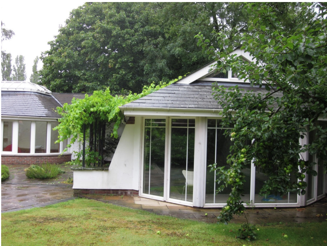
South elevation, conservatory and swimming pool enclosure
