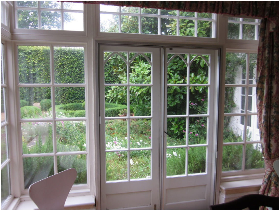
French windows from lounge, main house (facing west, service wing to right)
