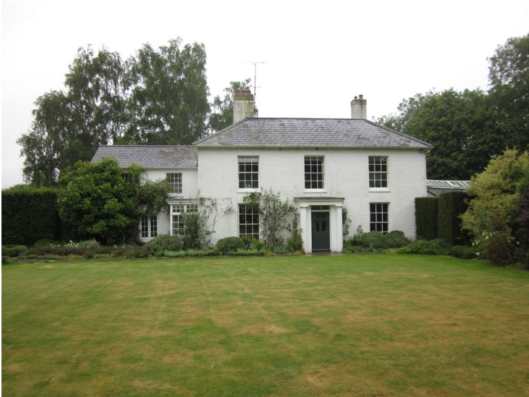
South elevation, main house and service (west) wing
